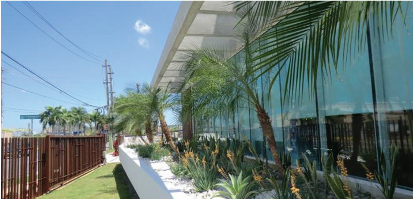
Coca-Cola Puerto Rico Yaucono Facilities Bayamón, Puerto Rico Ramírez Buxeda Arquitectos
